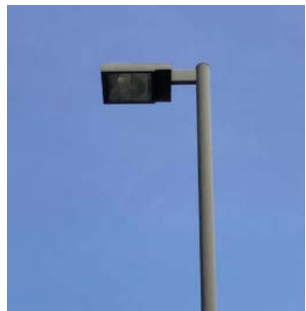
Pole Mounted HID Fixture
