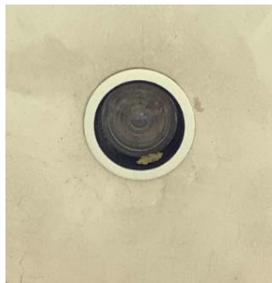
Ceiling Mounted CFL Lamp Fixture
